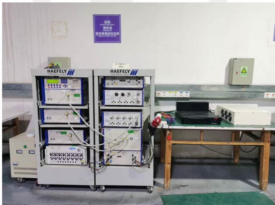
17.7.Photo of Surge Test
